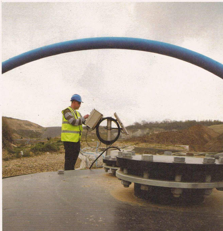
The remote monitoring of leachate, one area that OpenSpace is designed to help with
