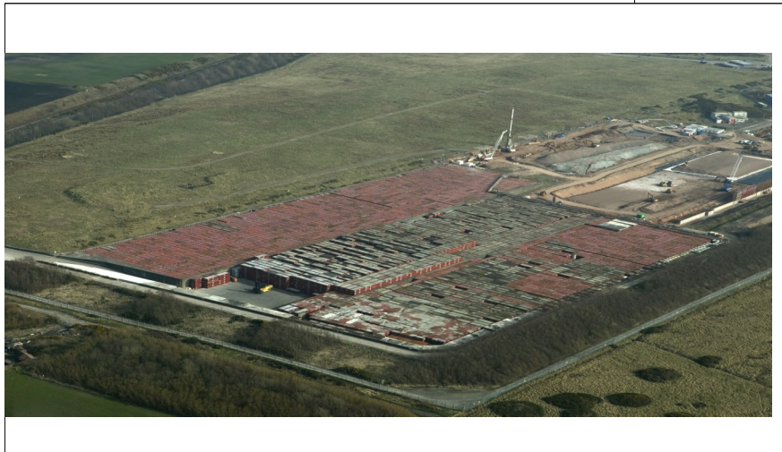
The low Level waste repository showing concrete vaults
